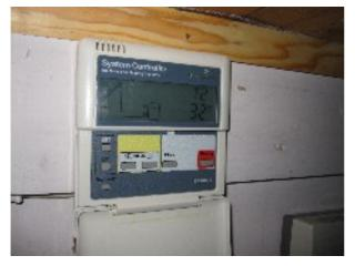
There's a control panel in the airing cupboard that records the temperature at the top of the panel, and at the top and bottom of the cylinder. Whenever the temperature at the top of the panel gets to 6 degrees higher than the water in the bottom of the cylinder the pump switches on, circulating an organic-based heat-transfer fluid.
